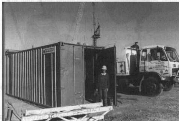
Joanne Green with the storage container from Container Rentals on the Sydney Olympics site.
