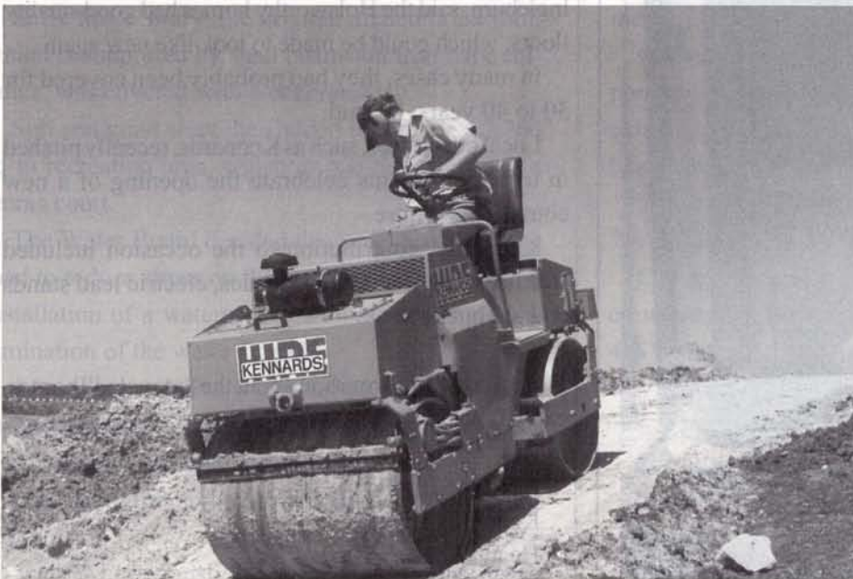
The Kennards' dual-drum roller which was used by Australian Native Landscapes at Cromwell Park.
