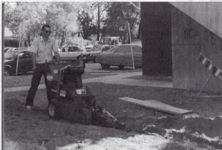
Tom Hawkins of Comtex Services uses the Kennards trenches at the Prince of Wales Hospital
