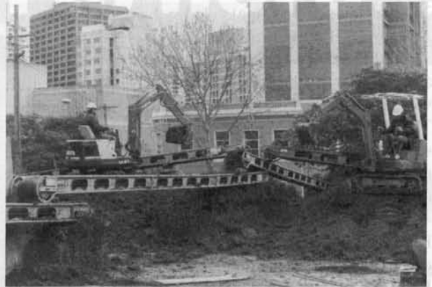
Two mini excavators load soil and grass on to linked portable conveyors on top of the Crown Street Reservoir
