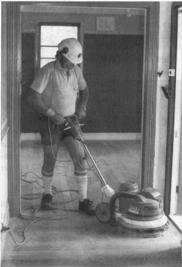
Nick Crisci of Twin Bros Floor Sanding uses the Kennards rotary sander on a former Army home at Holsworthy
